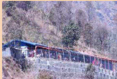
Kalidevi BS, Barabise-7 Truss modules I & II
